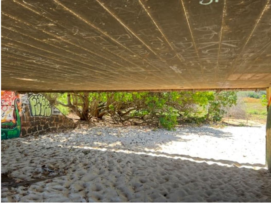
View from under existing bridge to location of new bridge.
