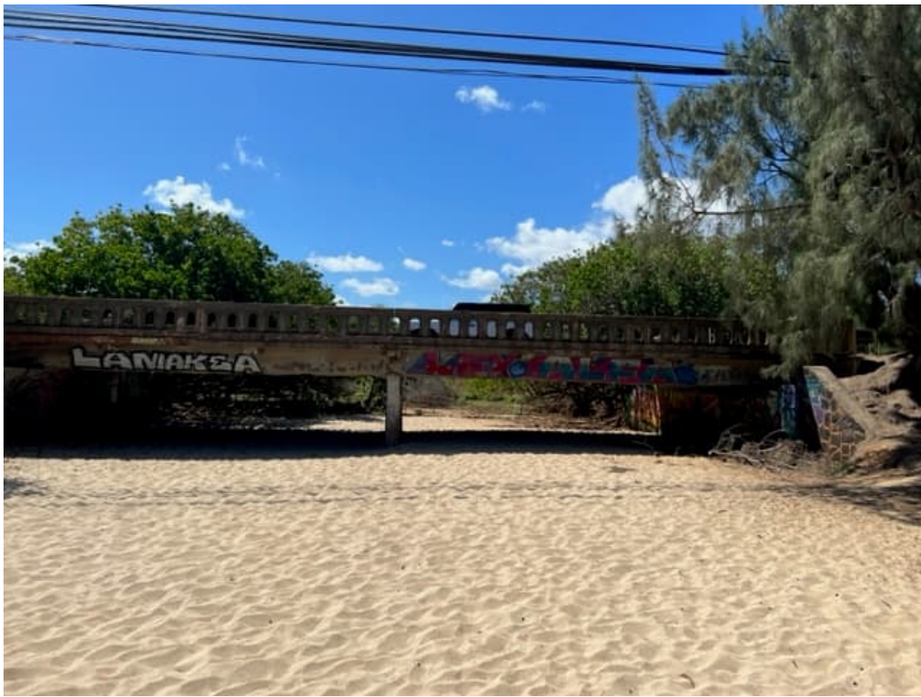
View of existing bridge from beach.
